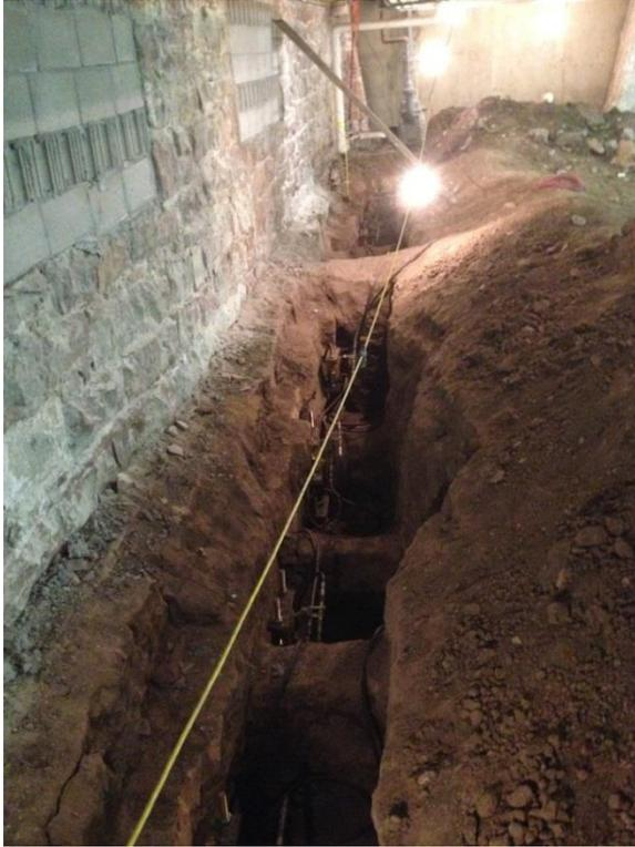
On the interior, the concrete slab in the basement was removed along the perimeter, holes were hand dug at the location of each pier and the footing was prepared to accept the bracket, ram and lift cylinder.
