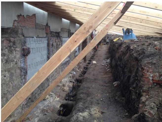
The exterior of the foundation was excavated to a depth of approximately 15' and a temporary shelter was built to keep the area heated and protected from the elements. During excavation, glass windows were removed and blocked in and footing preparation was started. At the location of each pier a hole was hand dug to gain access to the bottom of the footing, and the footing was chipped smooth to allow installation of the bracket and hydraulics.
