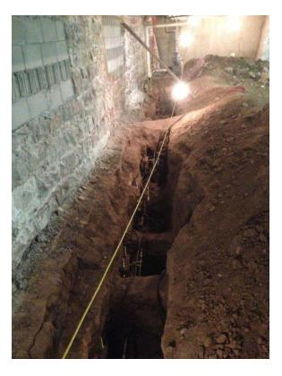
On the interior, the concrete slab in the basement was removed along the perimeter. Holes were dug by hand at the location of each pier and the footing was prepared to accept the bracket, ram and lift cylinder.
