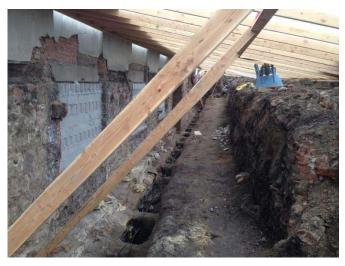
The exterior of the foundation was excavated to a depth of approximately 15 feet, and a temporary shelter was built to keep the area heated and protected from the elements. During excavation, glass windows were removed and blocked in and footing preparation was started. At the location of each pier, a hole was dug by hand to gain access to the bottom of the footing, and the footing was chipped smooth to allow installation of the bracket and hydraulics.
