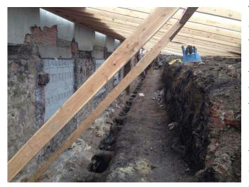
The exterior of the foundation was excavated to a depth of approximately 15 feet, and a temporary shelter was built to keep the area heated and protected from the elements. During excavation, glass windows were removed and blocked in and footing preparation was started. At the location of each pier, a hole was dug by hand to gain access to the bottom of the footing, and the footing was chipped smooth to allow installation of the bracket and hydraulics.
